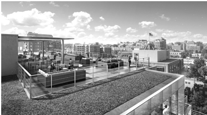
MTFA Architecture's 2311 Wilson Boulevard
