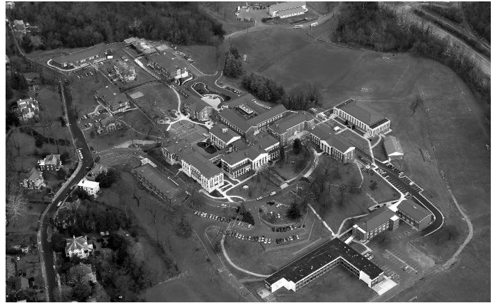
HENRY ADAMS Awarded VSDB Arc Flash Study Photo courtesy of VSDB
