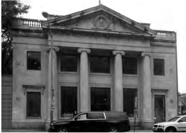
Embassy of India Restoration | Washington, DC
