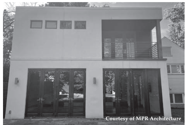
Rear façade before renovation.
