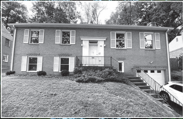
Front façade before renovation.
