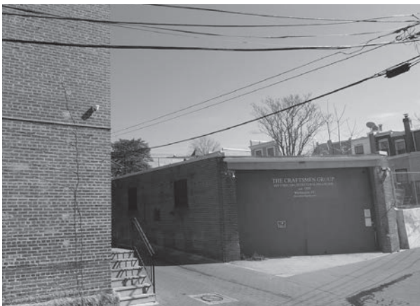
The building before the renovation and addition.
