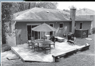
Rear patio before renovation. Courtesy of KUBE architecture
