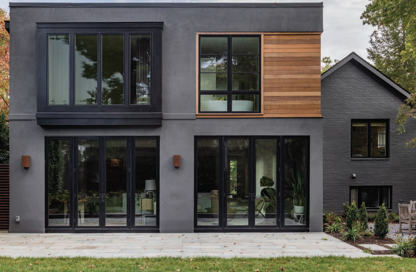
Rear façade with new bay window in the primary bedroom.
