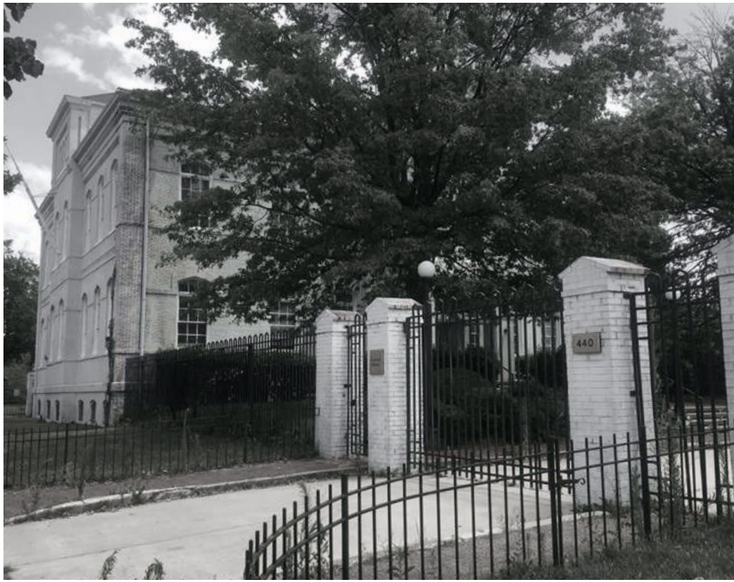
before and after, looking east along r street nw
