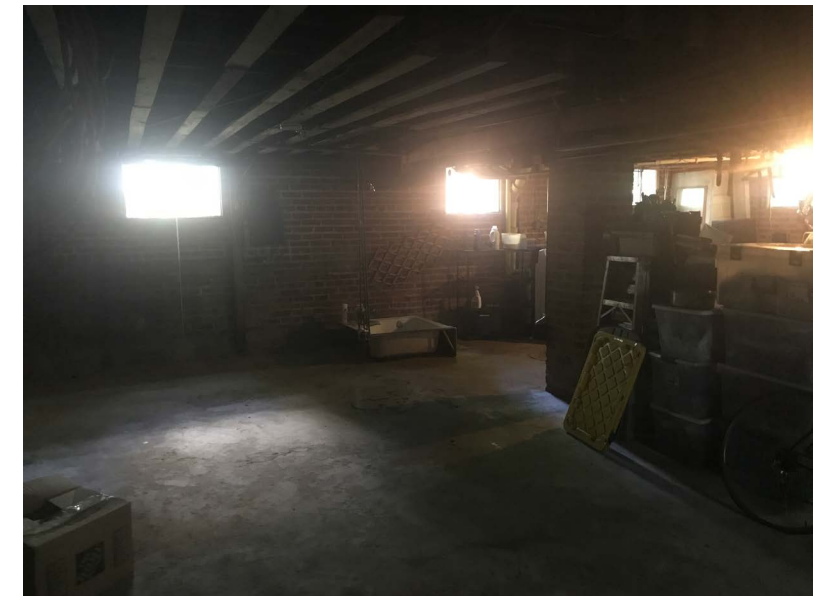
(above) basement before construction
