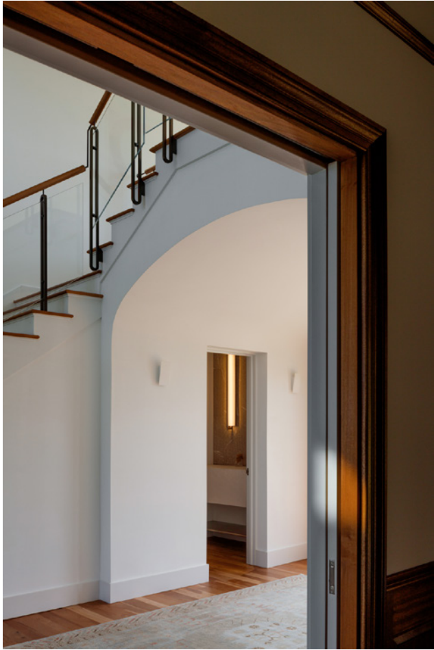
(above) The stair underside was sculpted to simplify geometries, and new glass rails opened views to the water.
