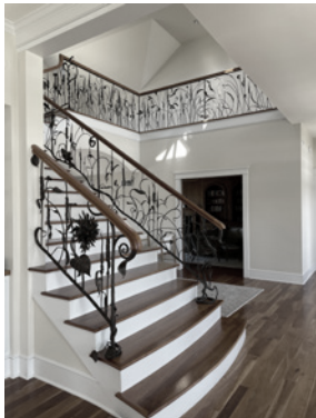
(right) Before view of stair hall with curved bottom treads and cast iron handrail. The handrail was repurposed as a new fence along the marsh grasses on the property.
