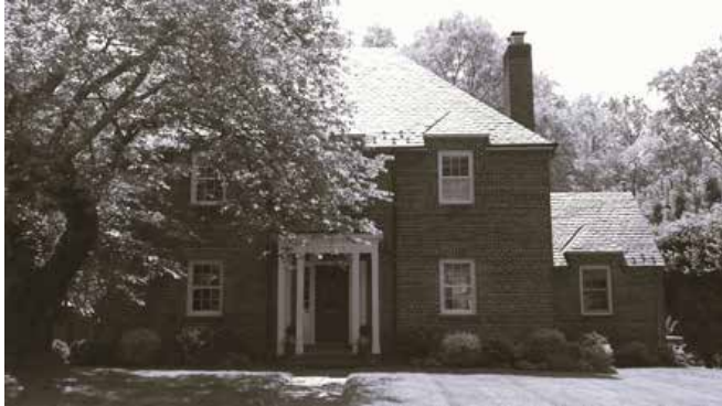
Before: North Elevation
