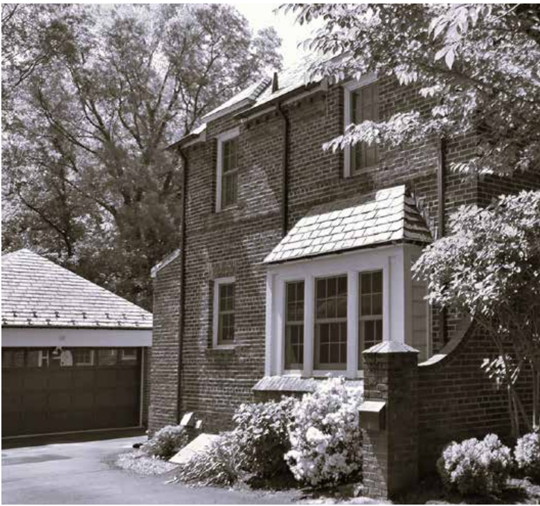
Before: East Elevation
