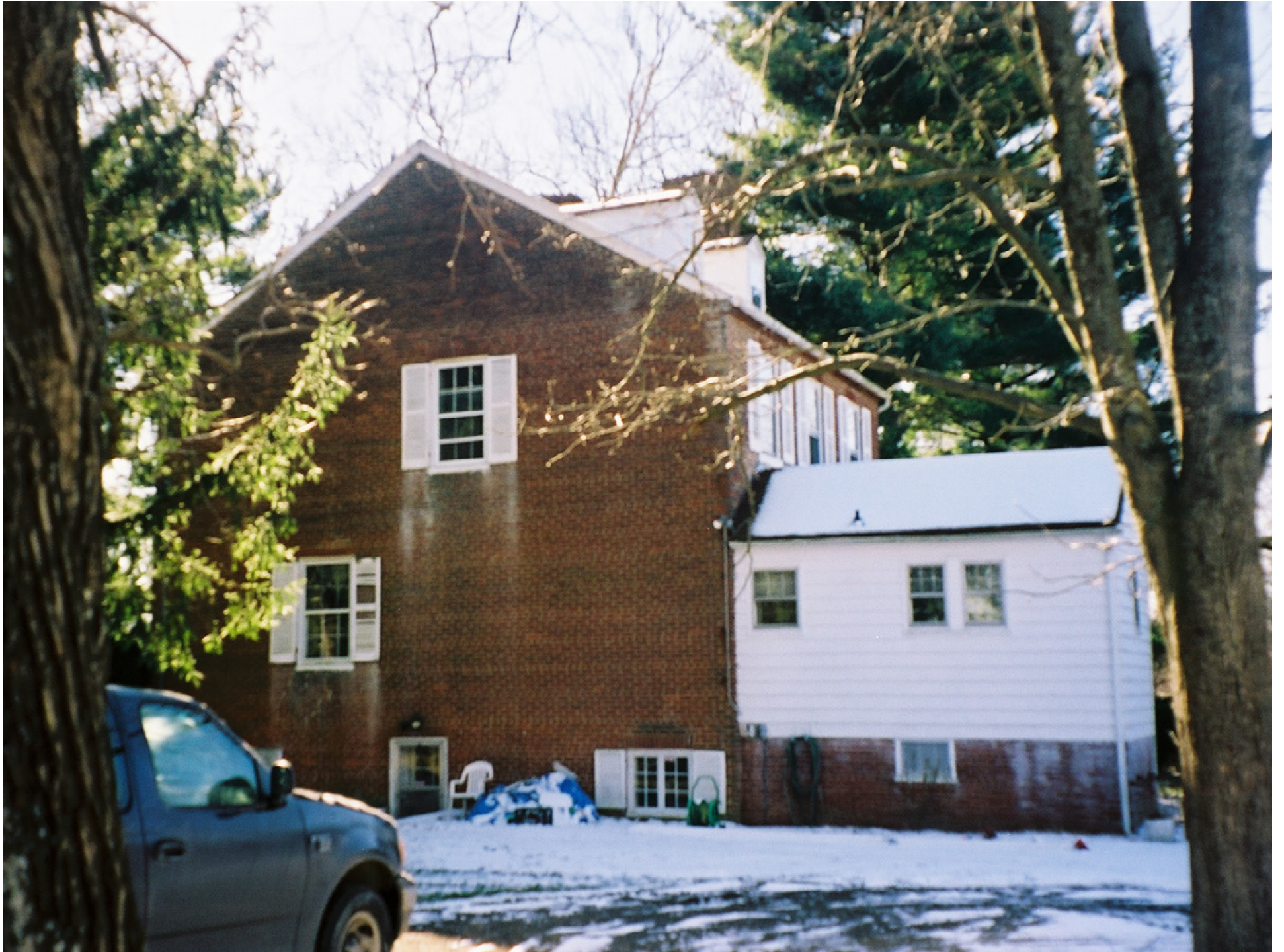
EXISTING EAST FACADE
