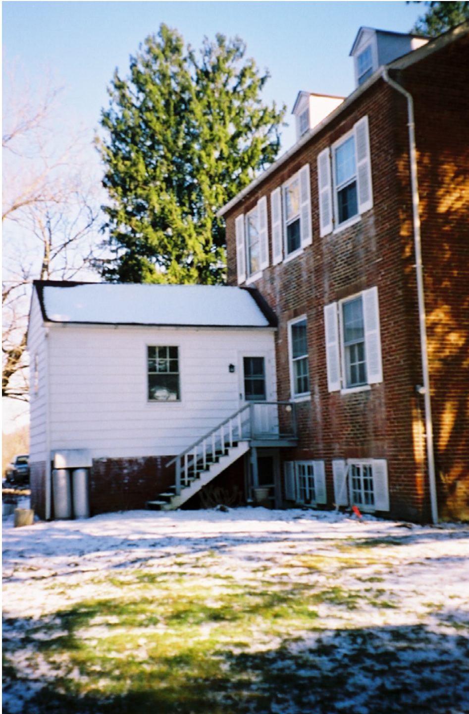
EXISTING WEST FACADE WITH KITCHEN
