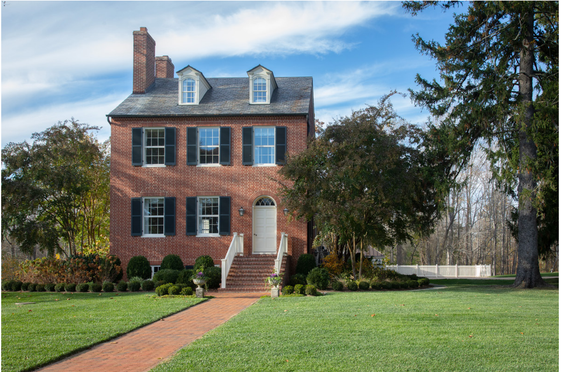
RESTORED SOUTH FACADE
