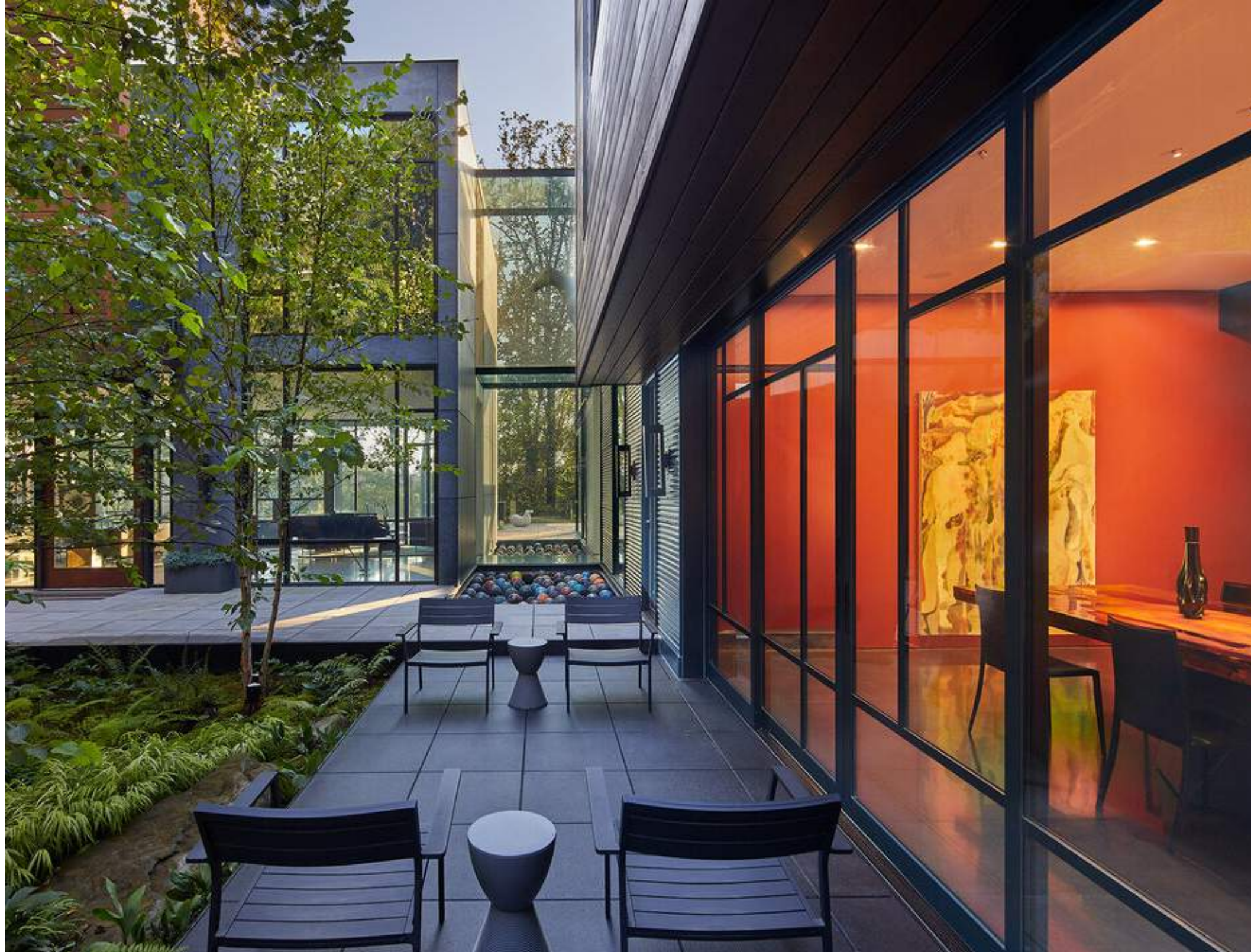
View from carport walkway across the new dining room patio toward the existing house. New dining room is visible on the right. A new window/door system has replaced the original garage doors.
