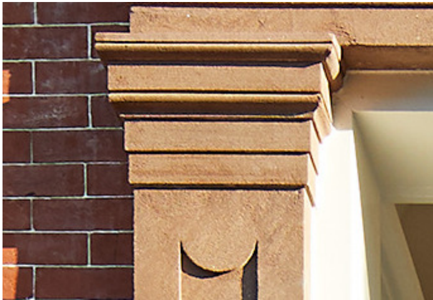
Restored Stone Detail 3
