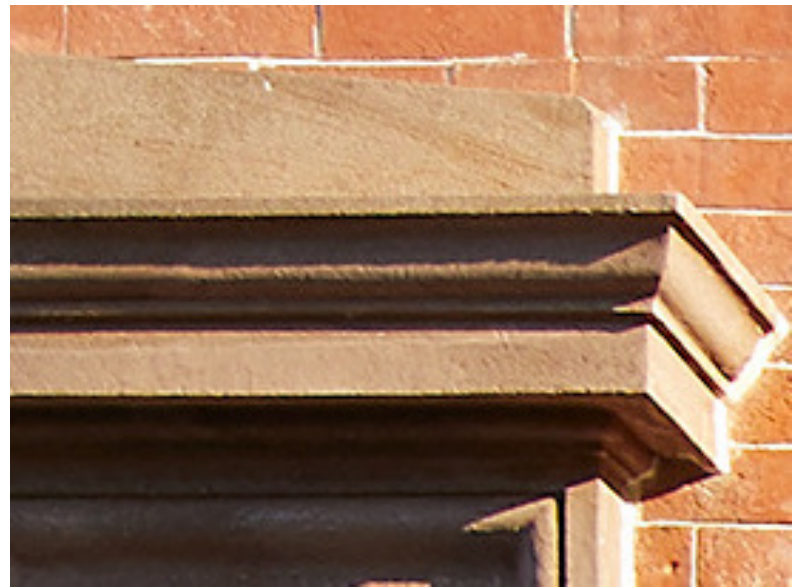
Restored Stone Detail 2
