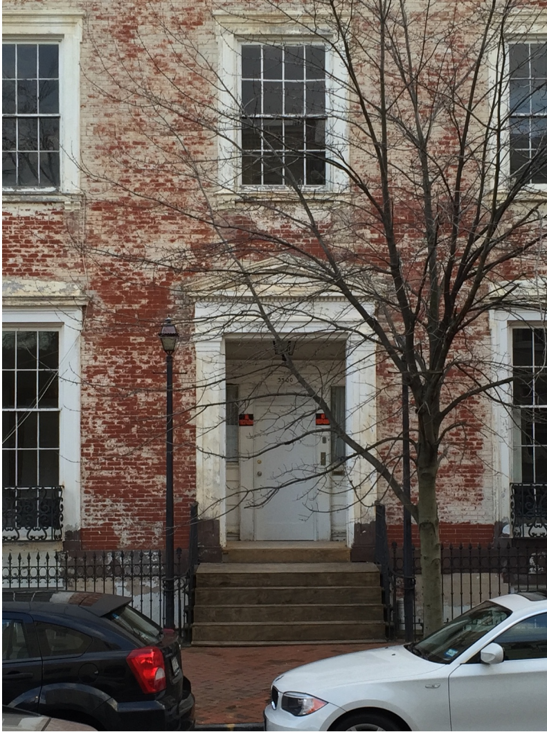
View of Entrance - Before
