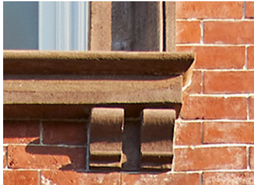
Restored Stone Detail 4
