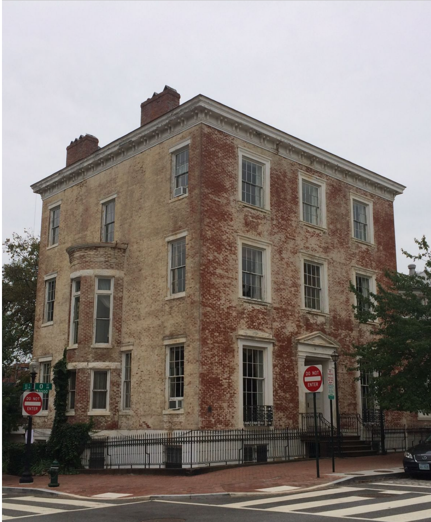
View From Northeast - Before
