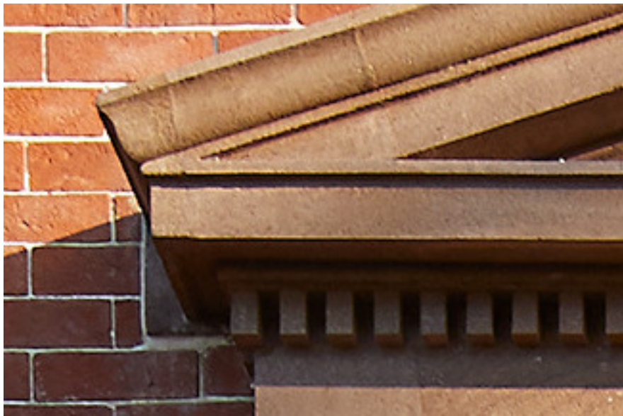
Restored Stone Detail 1
