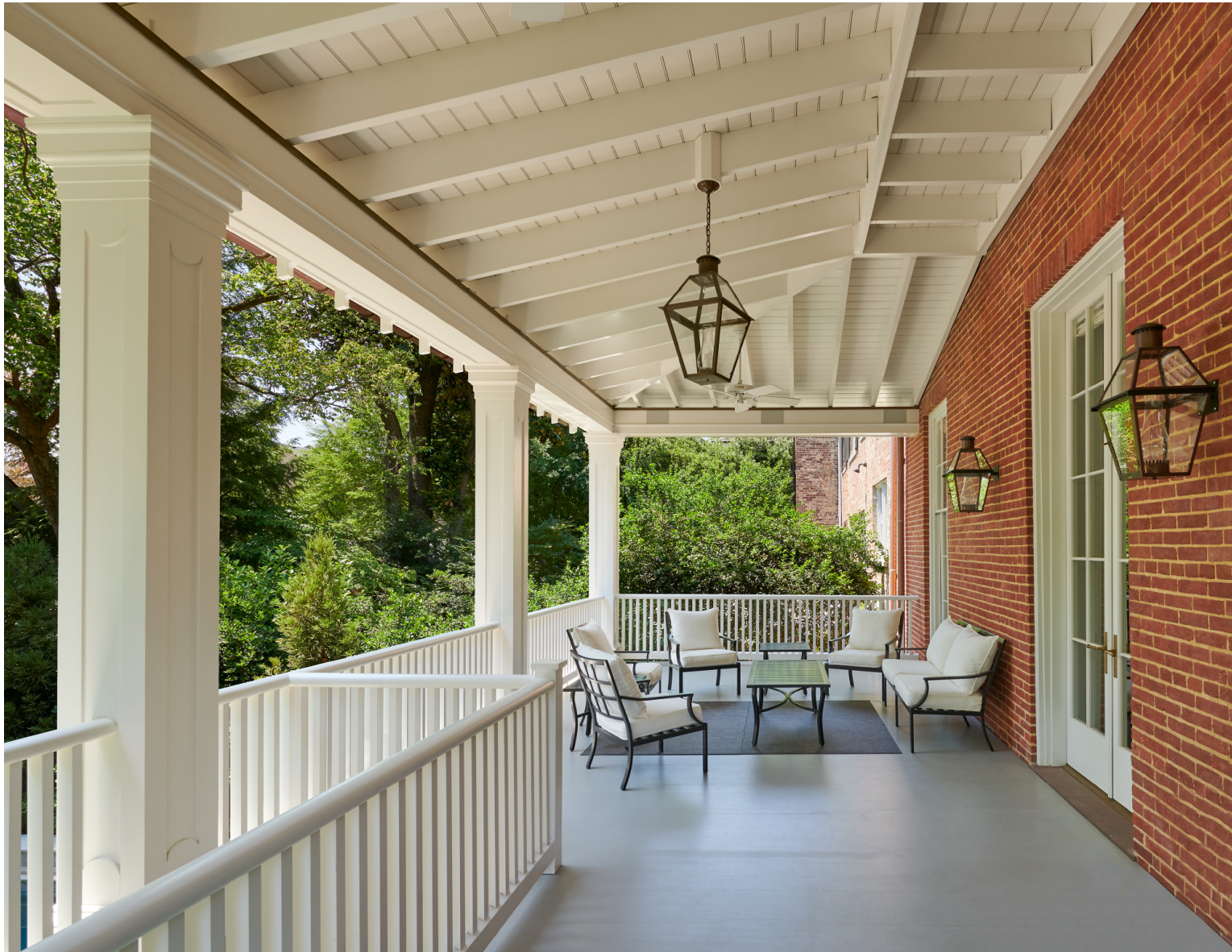
View of Porch Looking West
