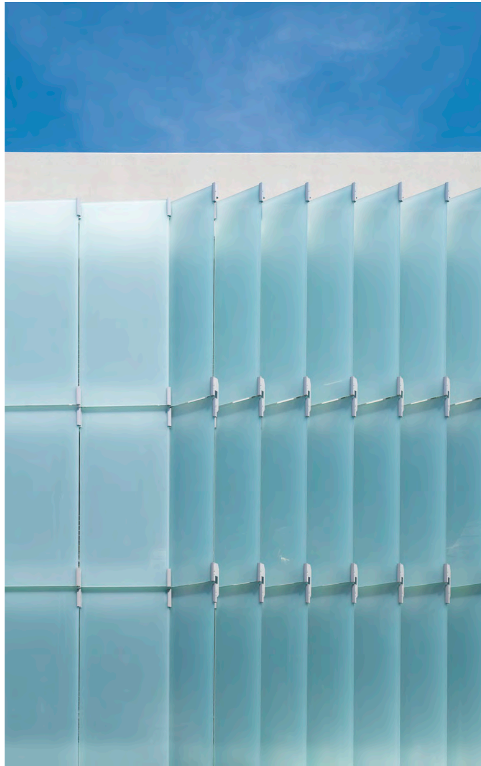
Shingle Glass - West Facade
