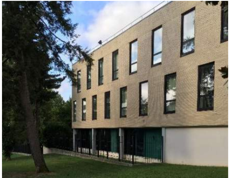
Office Wing, 1975 - 2004 Interventions
