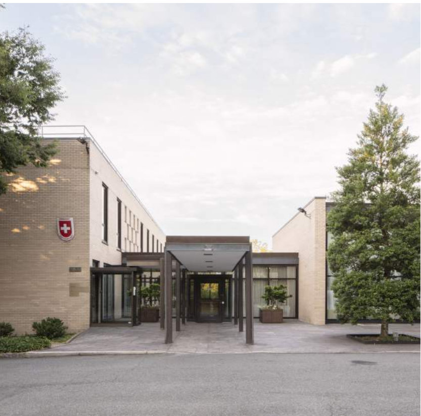
Entrance from Cathedral Avenue prior to Renovation
