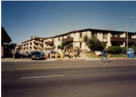
At the Northridge Meadows Apartments in Los Angeles, CA, the first story completely collapsed during the Northridge earthquake.
