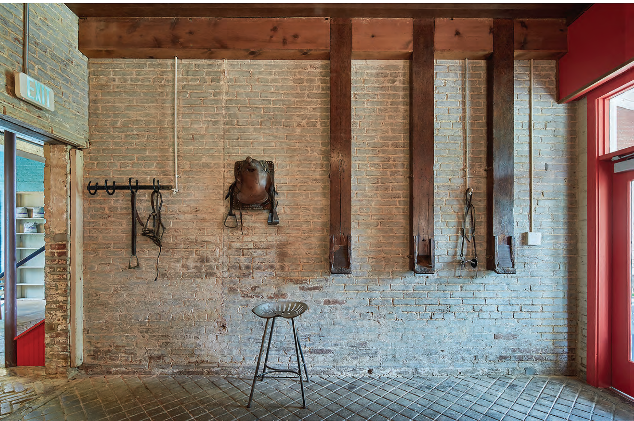
AFTER LOOKING WEST in 'FEED ROOM' - Scored concrete floor was preserved. High wood ceiling was preserved. Notice along the brick wall three historic grain chutes and two white painted gas pipes that still retain gas cocks (mid-to-late 19th century gas lighting).
