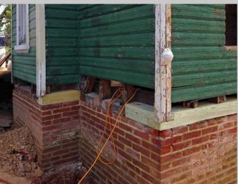
The original brick foundation received a thorough repointing and the original 6x6 sill plates were replaced. A new foundation at the rear of the house includes a veneer of salvaged brick found at the site. Composite shake roofing was used to replicate the original cedar shakes found under a deteriorated standing seam metal roof.
