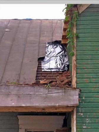
First task - stabilize the structure. Then, the architect carefully documented the many architectural features that remained - original reeded drop siding and decorative window dressings. Notable salvaged items include the only original window and its hardware at the front bay window and a louvered shutter at the side. The restorative process was a hand-in-hand effort between the architect, the contractor, and the Trust's development team including their in-house historic preservationist.
