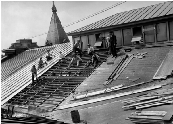
Historic Removal and replacement of Hall slate roof with metal standing seam, circa 1906-1908.
