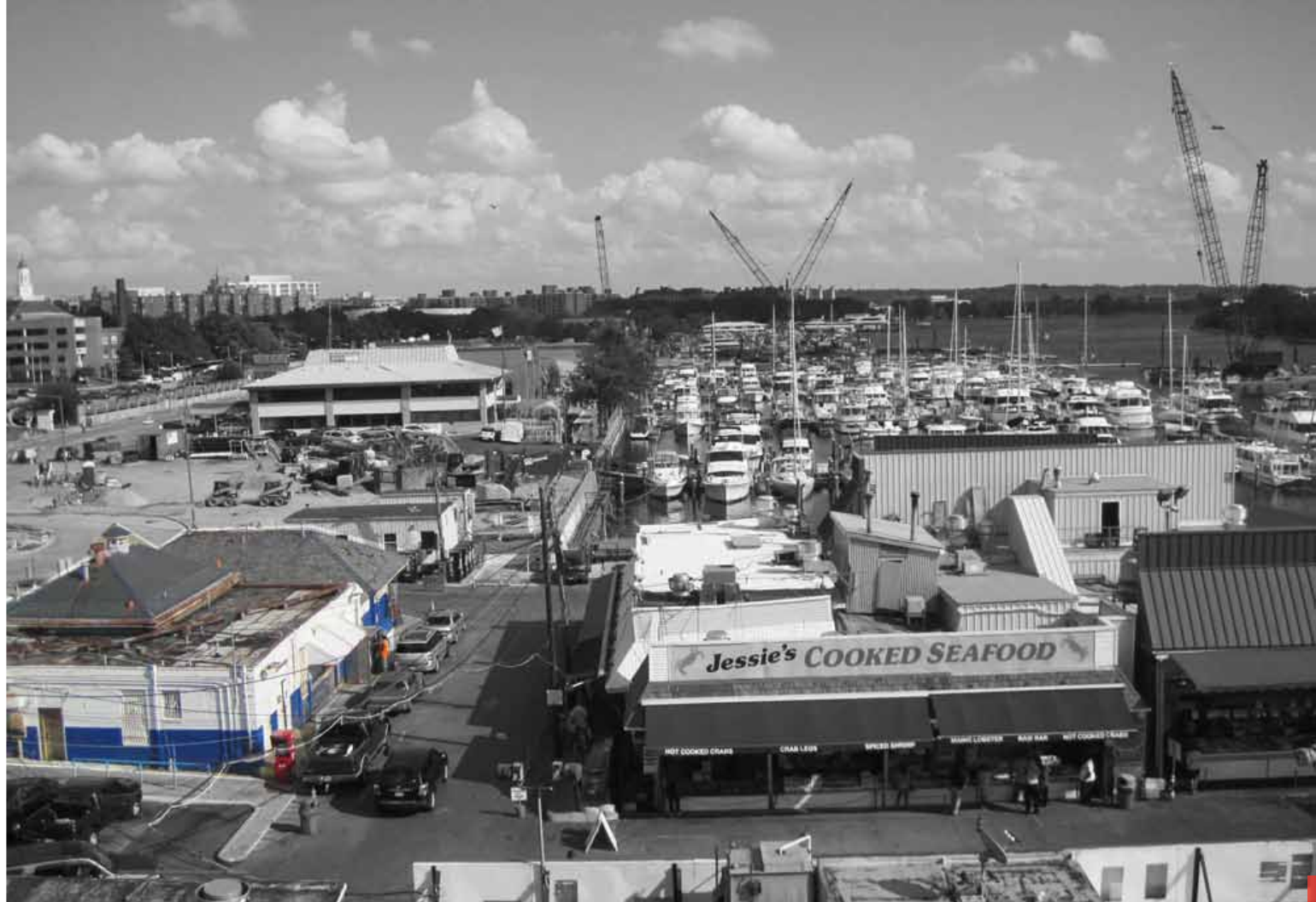
PRE-DEVELOPMENT SETTING OF HISTORIC LUNCH ROOM AND OYSTER SHED (SHOWN IN COLOR) WITH WHARF CONSTRUCTION IN THE BACKGROUND
