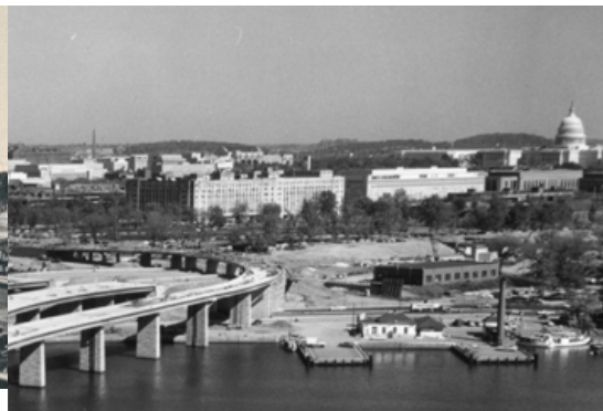
HIGHWAY CONSTRUCTION NEAR LUNCH ROOM, SHED AND UNDOCUMENTED SMOKESTACK 1961
