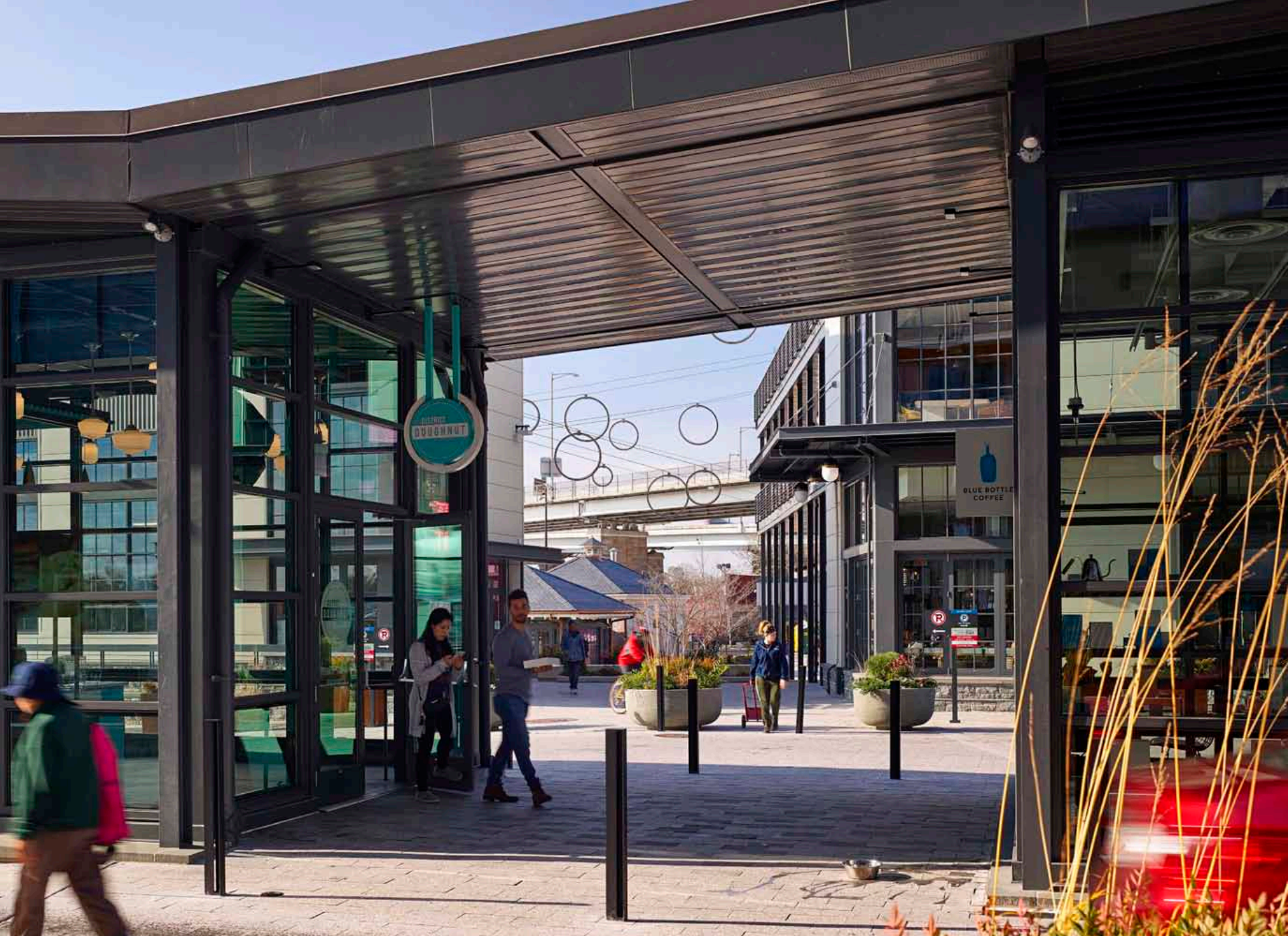
THE NEW MARKET SHED FRAMES A VIEW ACROSS MARKET SQUARE AND TOWARDS THE RENOVATED 1916 STRUCTURES
