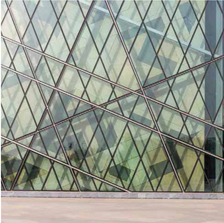
exterior | aluminum and steel cassette framing system for curtain wall ▲
