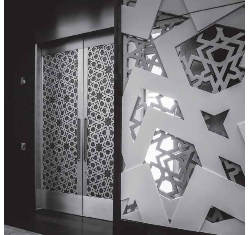
interior | mashrabiya panels of glass-reinforced gypsum ▲
