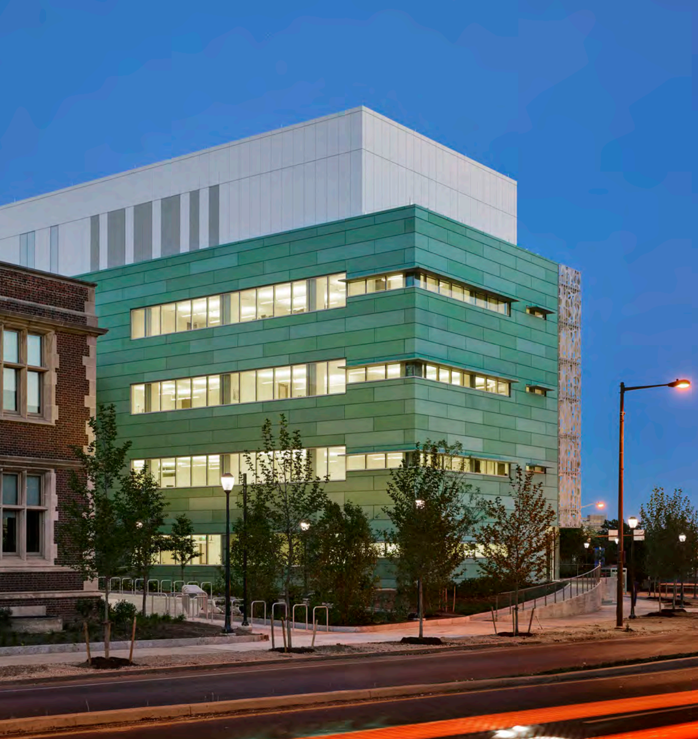
The copper volume contains the labs. Testing and rooms that need controlled light are located in the center of the space and graduate student workrooms are located at the perimeter where north-facing windows provide generous light.
