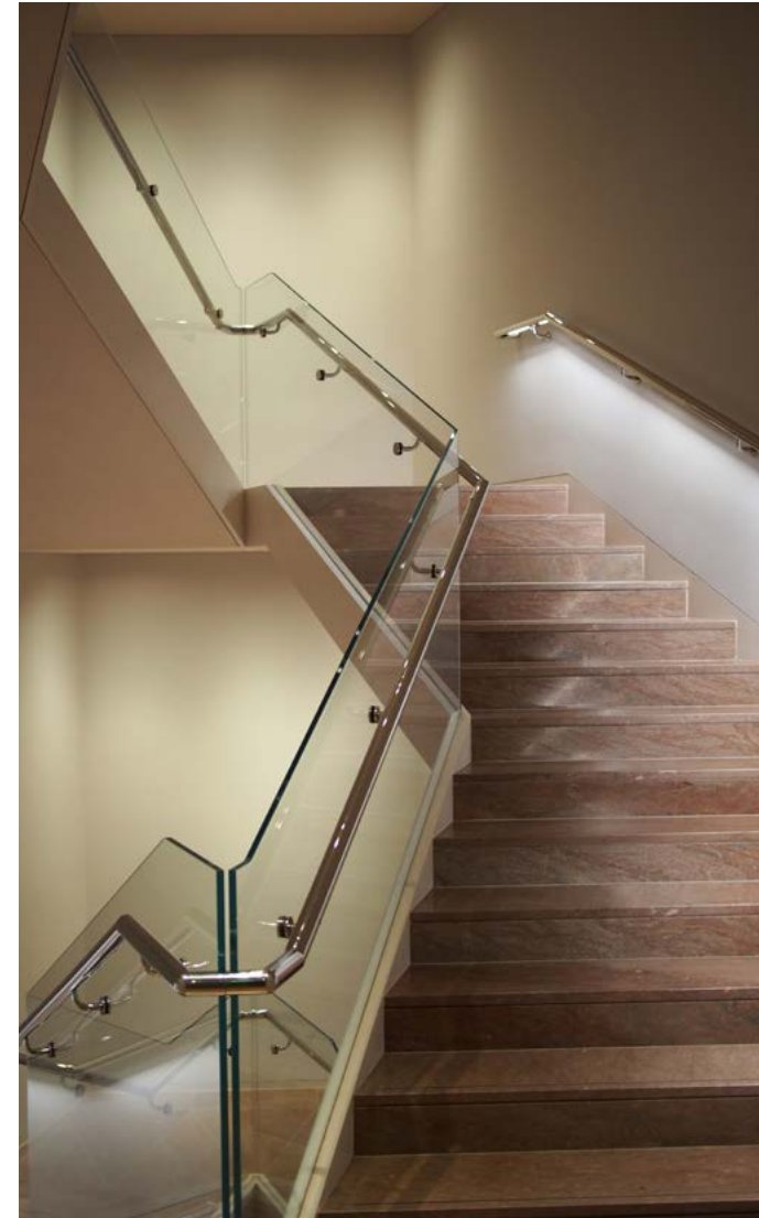
Final installation of stair
