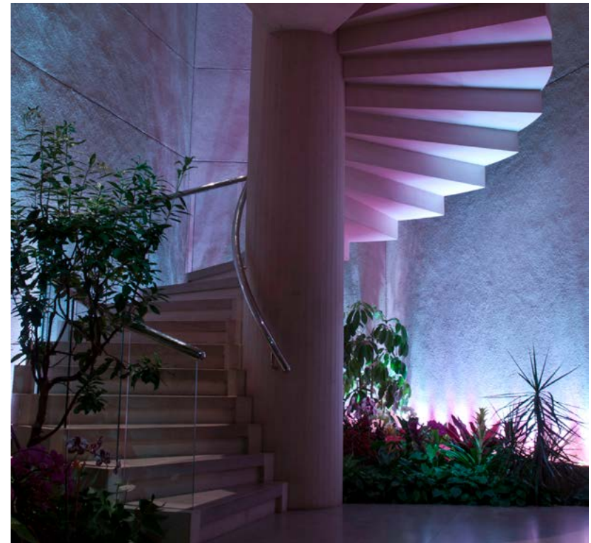
△ Existing spiral stairs were removed as they did not meet the necessary egress requirements
