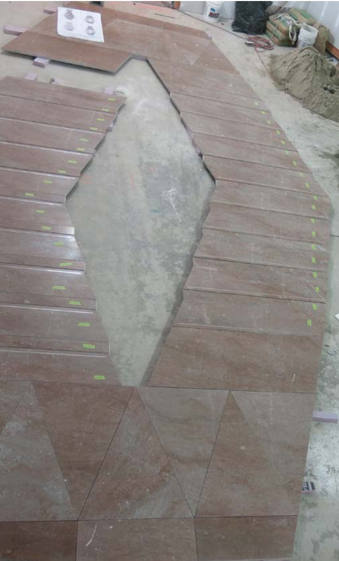
Dry-lay of Tennessee Pink Marble stair treads
