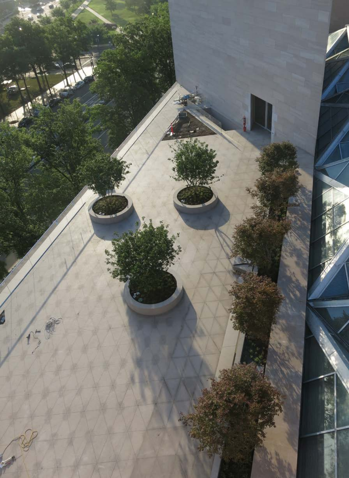
△ Existing ballast roof prior to the renovation/expansion project
