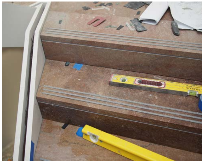
Mock-up and review of stair
